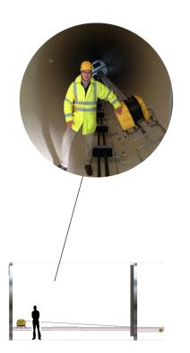
The Limpet® is bolted to the floor or back face of the ladder before the first section of turbine is erected and a pulley is fixed through the top ladder rungs of that section
